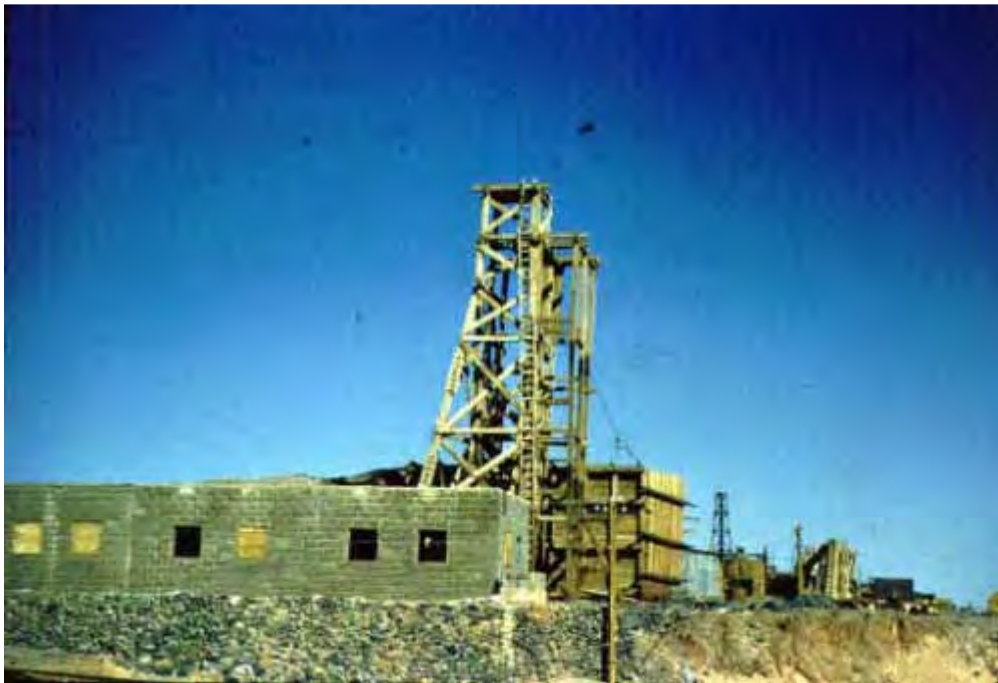
Zalim Mine Site Construction
