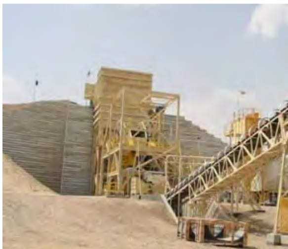
Processing Mill at Bulghah Mine
